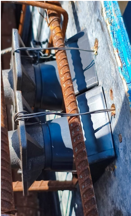
INSTALLED ON THE FORM
